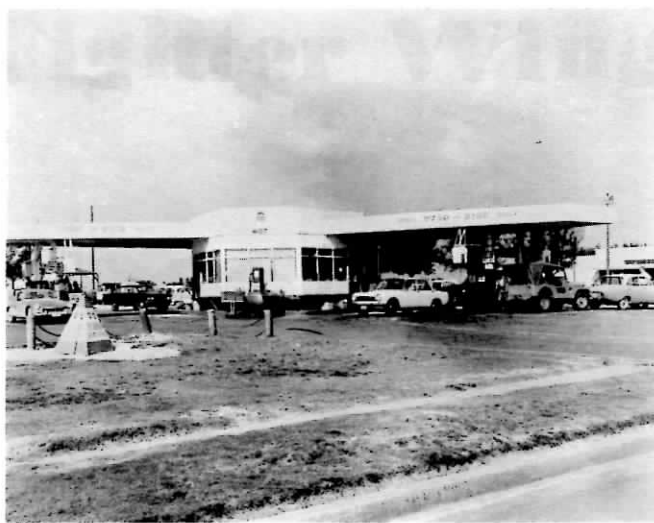
A typical on base service station.
