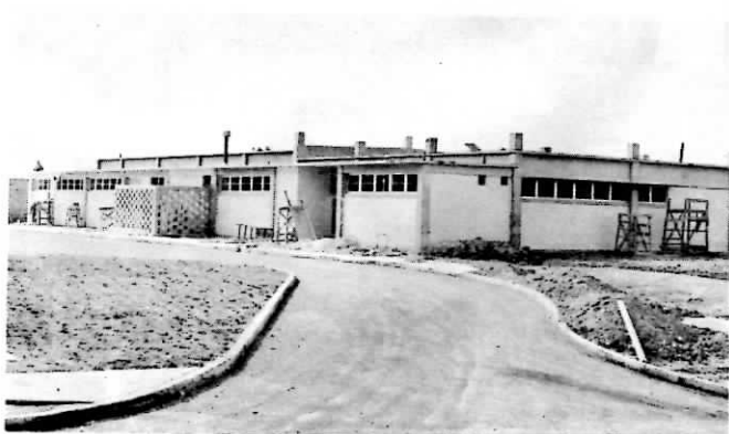
Early Progress On The New Service Club
