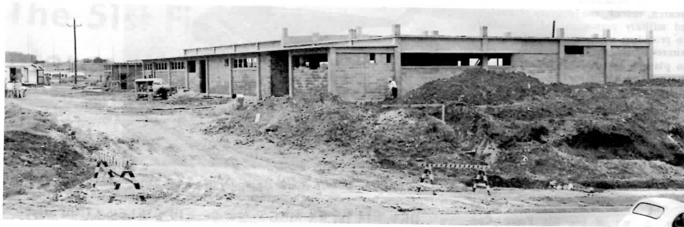
Construction Almost Completed On New Service Club
