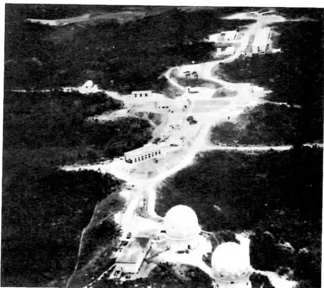
One of Four 51st FIW Radar Sites
