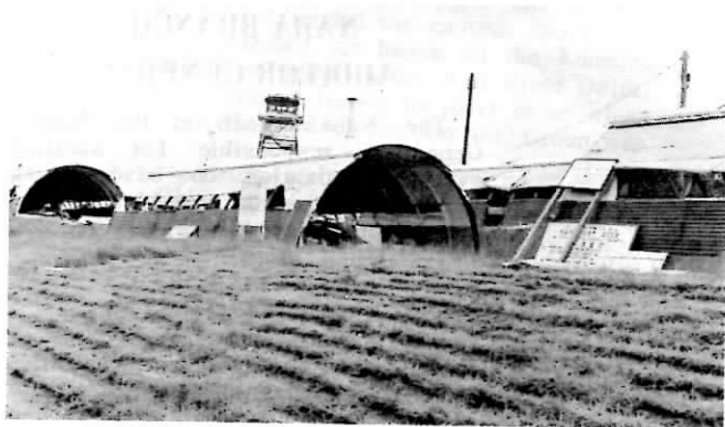
Quonset Buildings Being Torn Down
