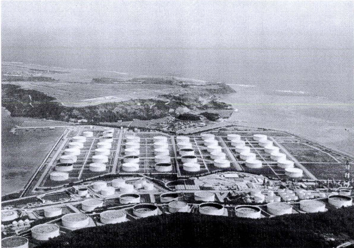
Figure 5. After Ocean Reclamation and the CTS Construction
